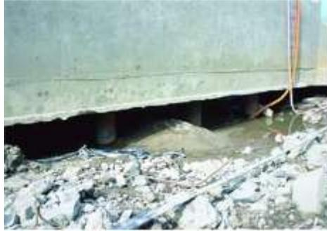
Fig. 1 Cavity development and embankment collapse (Kim 2014)
