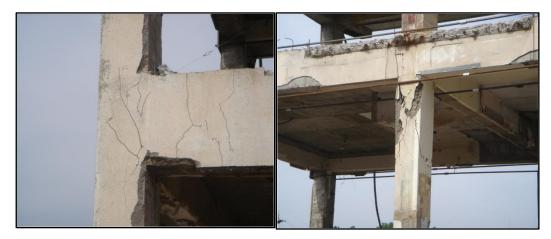
Fig.7 Crack of exterior beam-column jointFig.8Central columnfailure
