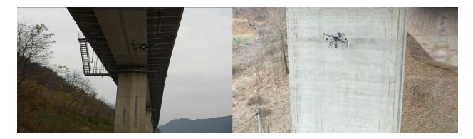
Fig. 1 Macro inspection using non-contact type UAV and micro inspection using contact type UAV
