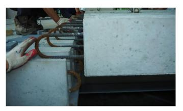
Fig. 3 Precast deck system allowing vertical installation
