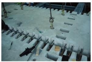
Fig. 2 Connection of precast deck with ribbed loop reinforcement
