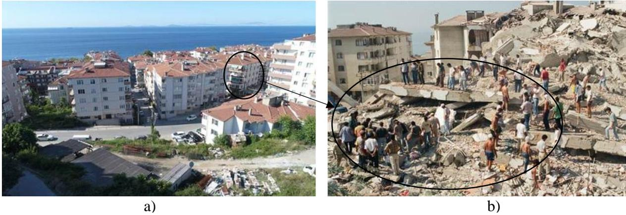
Fig. 2 Before and b) after views of collapsed RC structure.
